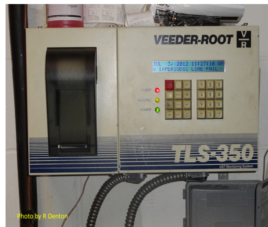
Automatic Tank Gauge showing failure (Photograph by Richard Denton)
